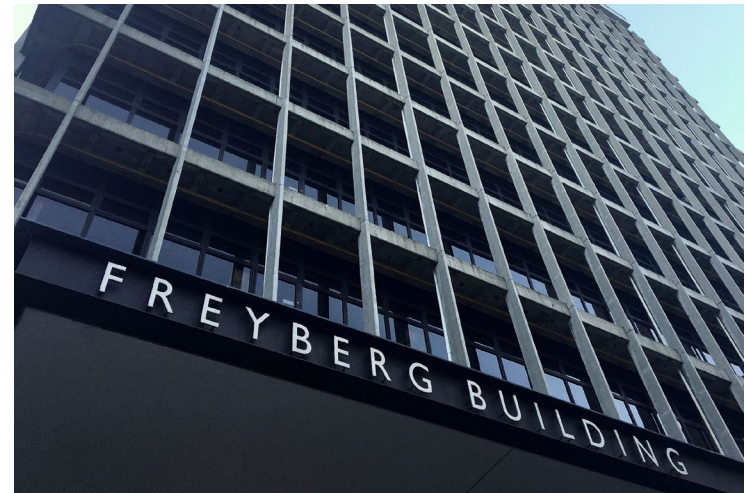
Freyberg Building - Key metrics
